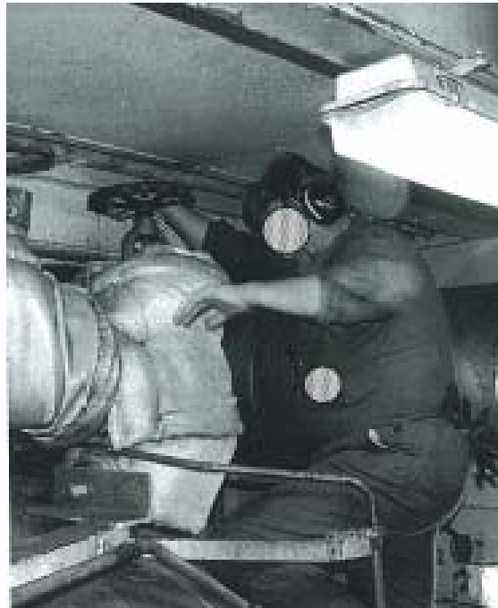
Fig. 3.17.1 Poor installed direction of valve
