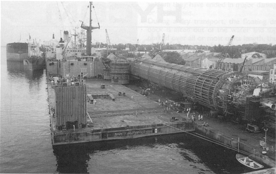
Fig. 7. Skidding-on of the Challis Field SALRAM.
